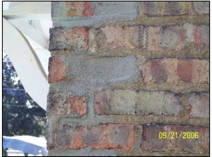
Previously repaired areas
