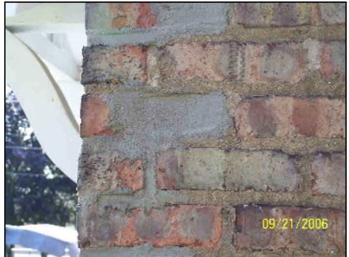
Previously repaired areas
